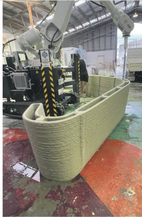
3D printing trials with QOROX in Hamilton. It's 75% faster and reduces waste by 70% when compared to traditional construction.
